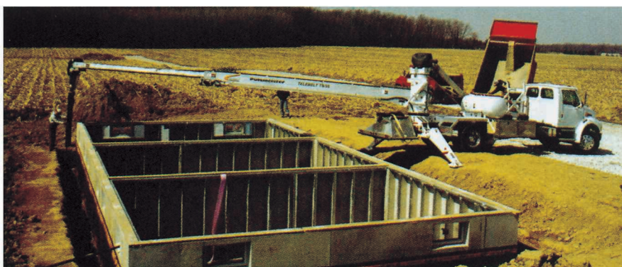
Conveyors place volumes of concrete, sand, and stone, creating a material handling value for contractors who want to expand operations and reduce reliance on other contractors.
